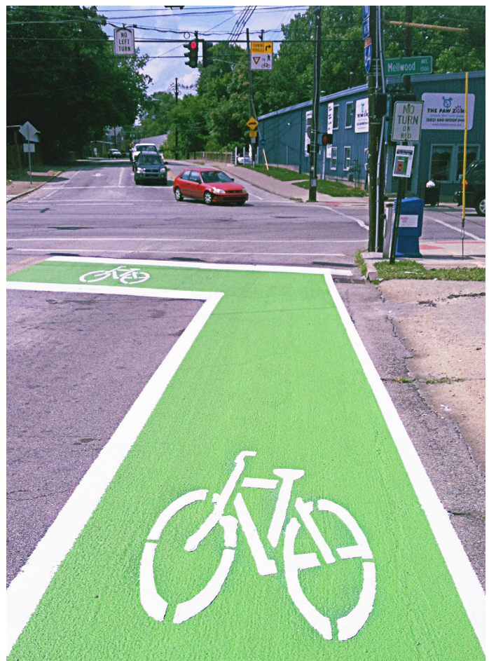
Louisville, Ky., installed a color pavement marking system on a number of bike lanes. (Photo courtesy of Transpo Industries)
